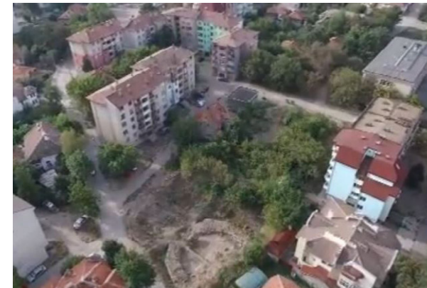
The ruins of the decagonal Roman tower from Bononia are found in the midst of a residential quarter in Bulgaria's Vidin
